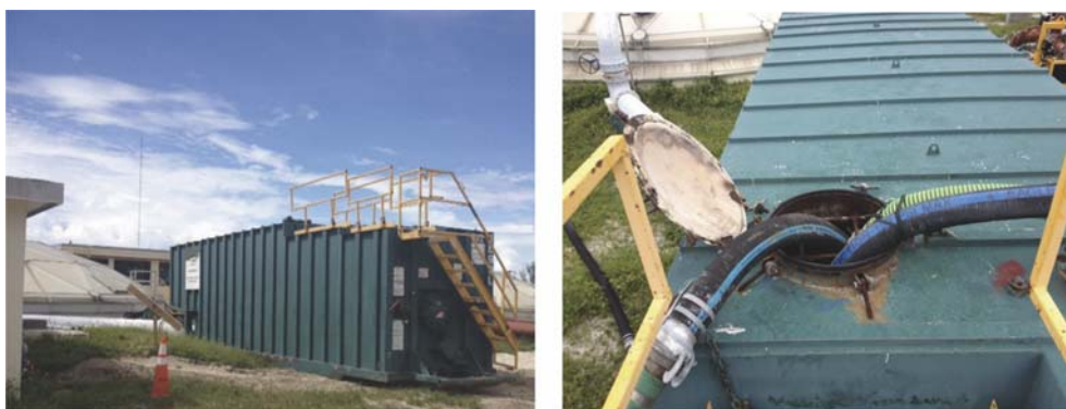
Figure 6. Central District Wastewater Treatment Plant and North District Wastewater Treatment Plant Blend Tank
