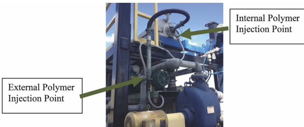
Figure 3. Thickening Polymer Injection Point
