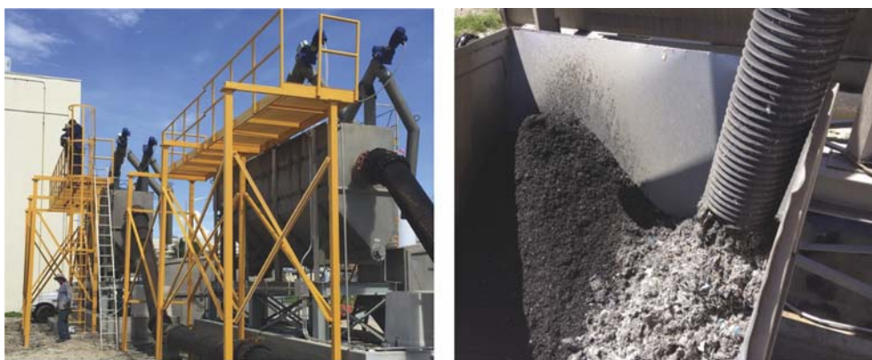
Figure 5. Central District Wastewater Treatment Plant Screens for North District Wastewater Treatment Plant Sludge
